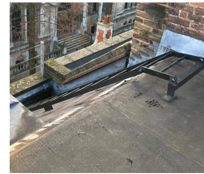
Figure 30: Condemned Roof Access Ladder
