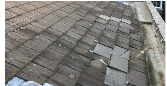
Figure 39: Existing Slates to Shallow Pitch
