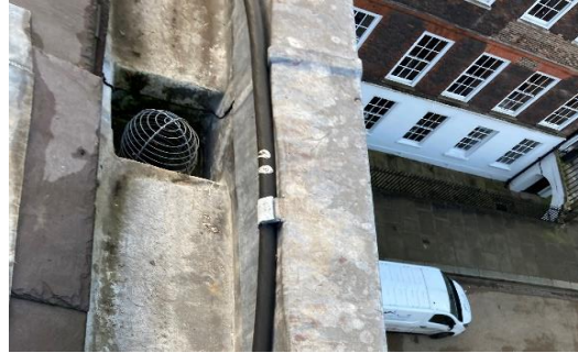
Figure 38: Broken Lead Cable Welt
