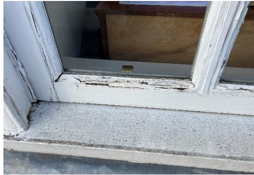
Figure 14: Defective Timber Sash Windows
