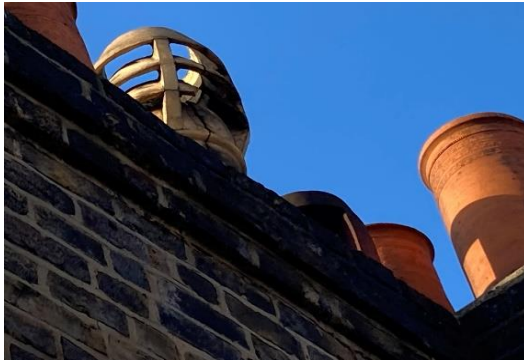
Figure 19: Cracked Chimney Cowl
