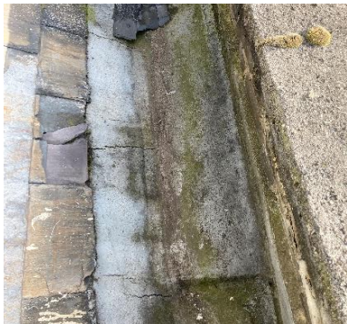
Figure 4: Parapet Gully (Rear)
