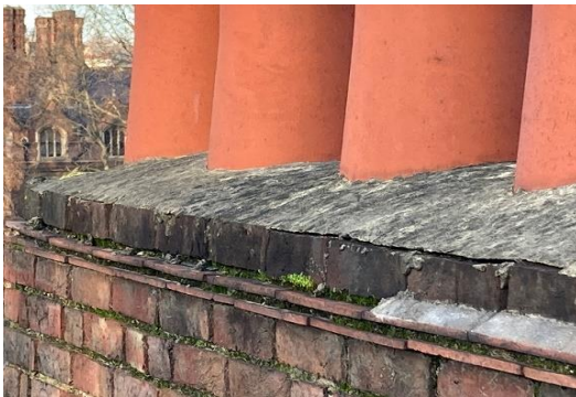
Figure 34: Defective Flaunching
