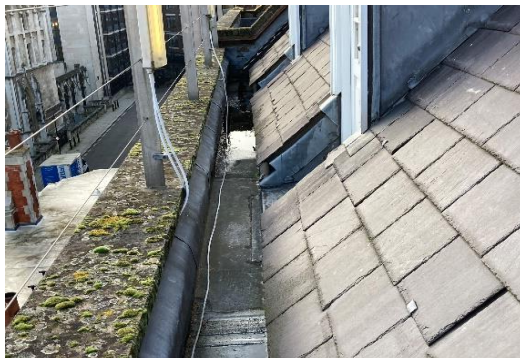
Figure 28: Existing Slates & Coping Stone
