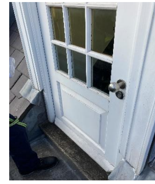
Figure 27: Defective Timber Weatherbar
