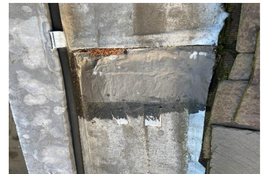
Figure 36: Flash Band Roof Repair
