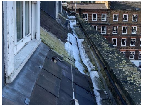
Figure 23: Parapet Gutter Front Elevation
