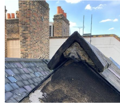
Figure 9: Loose Ridge Tile
