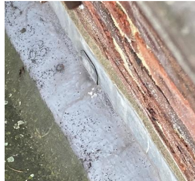
Figure 41: Acropol Repairs to Flat Roof
