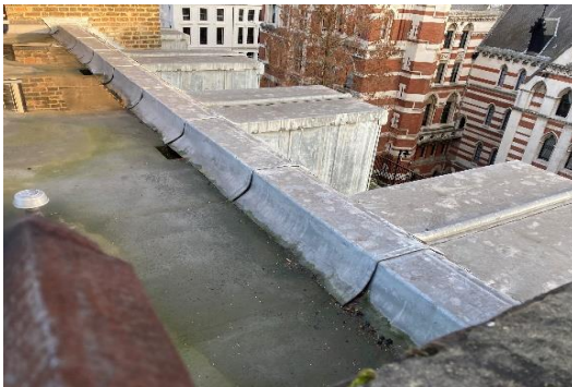
Figure 40: Leadwork to Dormers (Rear)
