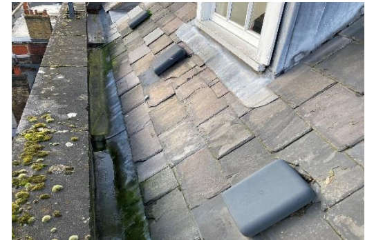
Figure 18: Existing Plastic Roof Vents
