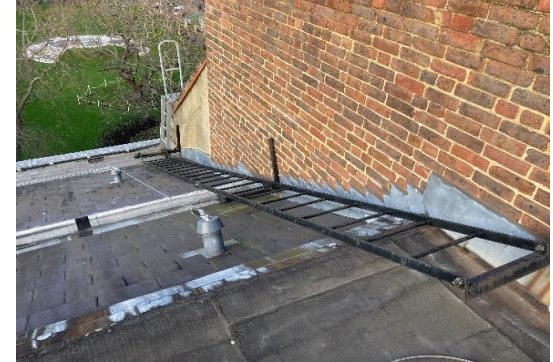
Figure 33: Condemned Roof Access Ladder
