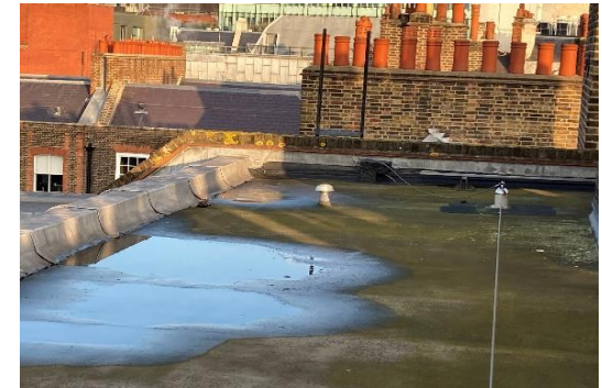
Figure 42: Ponding Water on Flat Roof
