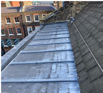
Figure 10: Lead Bays (Front)
