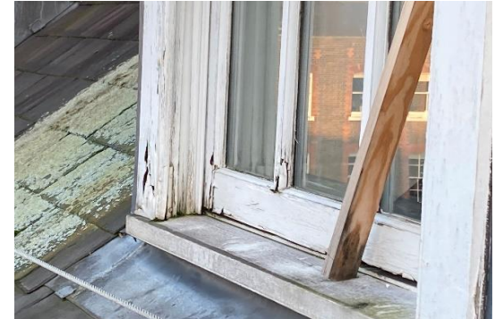
Figure 15: Defective Timber Sash Windows
