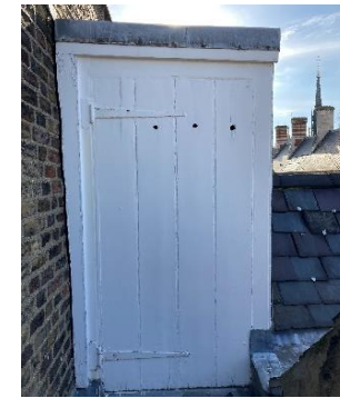
Figure 12: Painted Shut Roof Access Door
