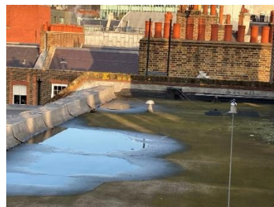
Figure 5: Existing Felt Roof 6 New Square
