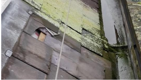
Image 5: Existing Roof Construction
