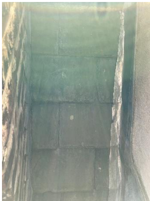
Image 8: Flashband Repair to Flashing
