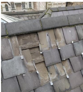
Image 4: 5 New Square East Pitched Roof Section
