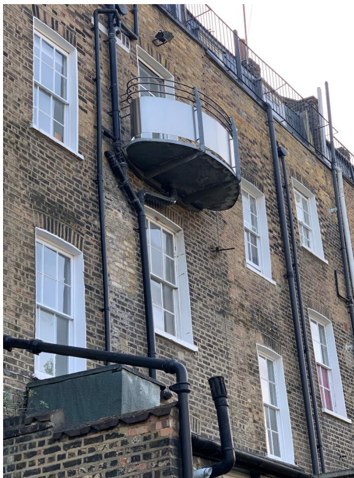
Figure 5: Rear elevation of 26 Mornington Terrace
