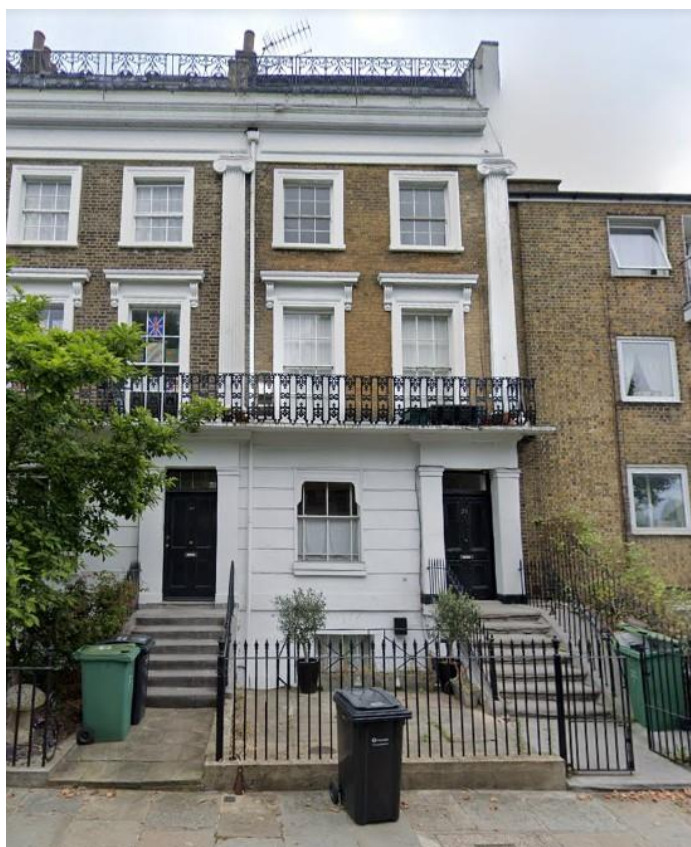
Figure 4: Principal façade of 26 Mornington Terrace
