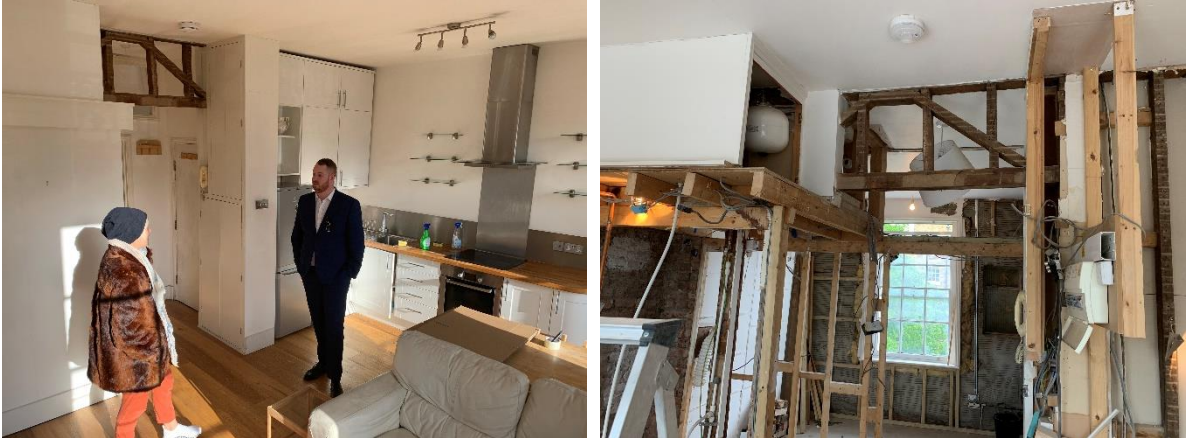
Figure 9: The timber stud frame (pre-existing) and during removal
