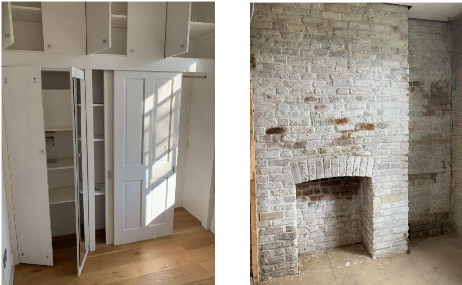
Figure 11: Pre-existing built-in cupboard in rear room and restored fireplace after removal of the cupboard
