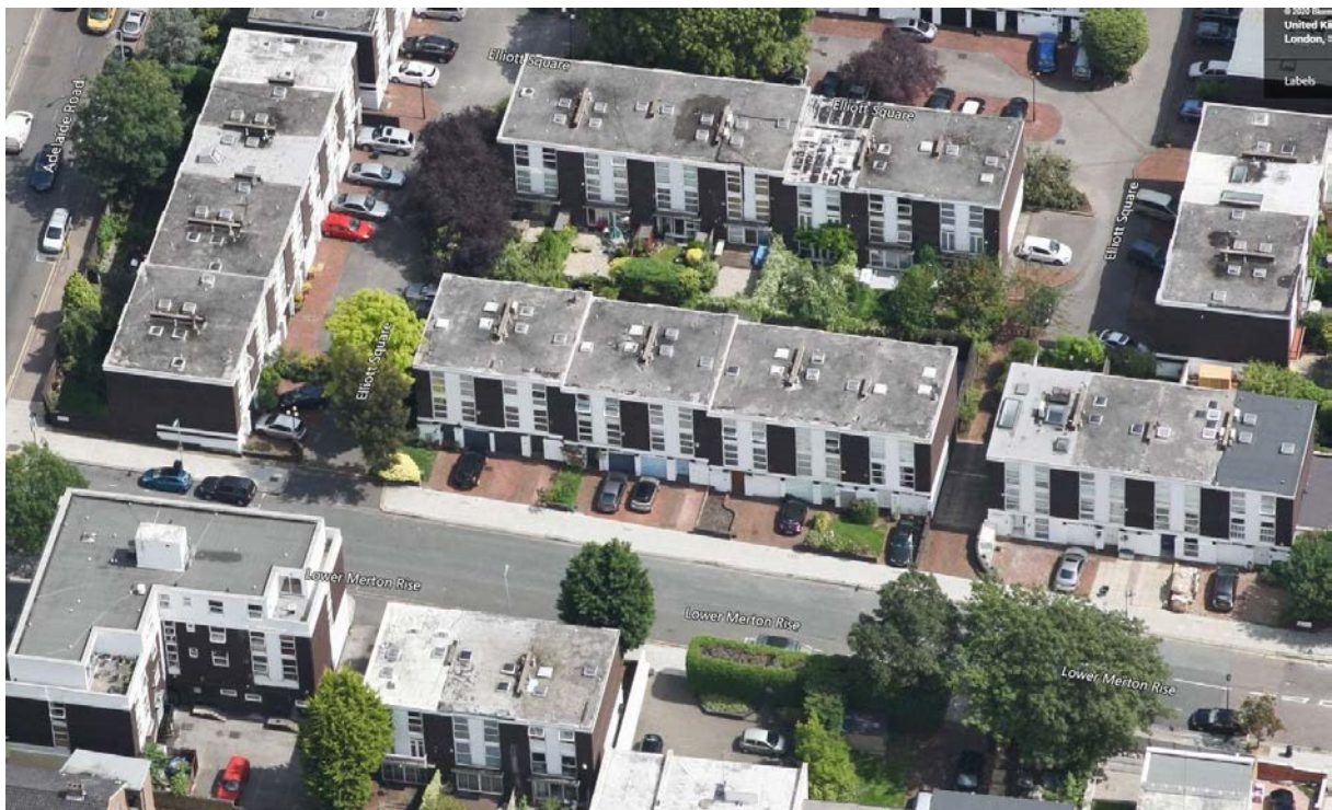
Figure 1 - Aerial photo of the site and surrounding buildings (©Bing)
