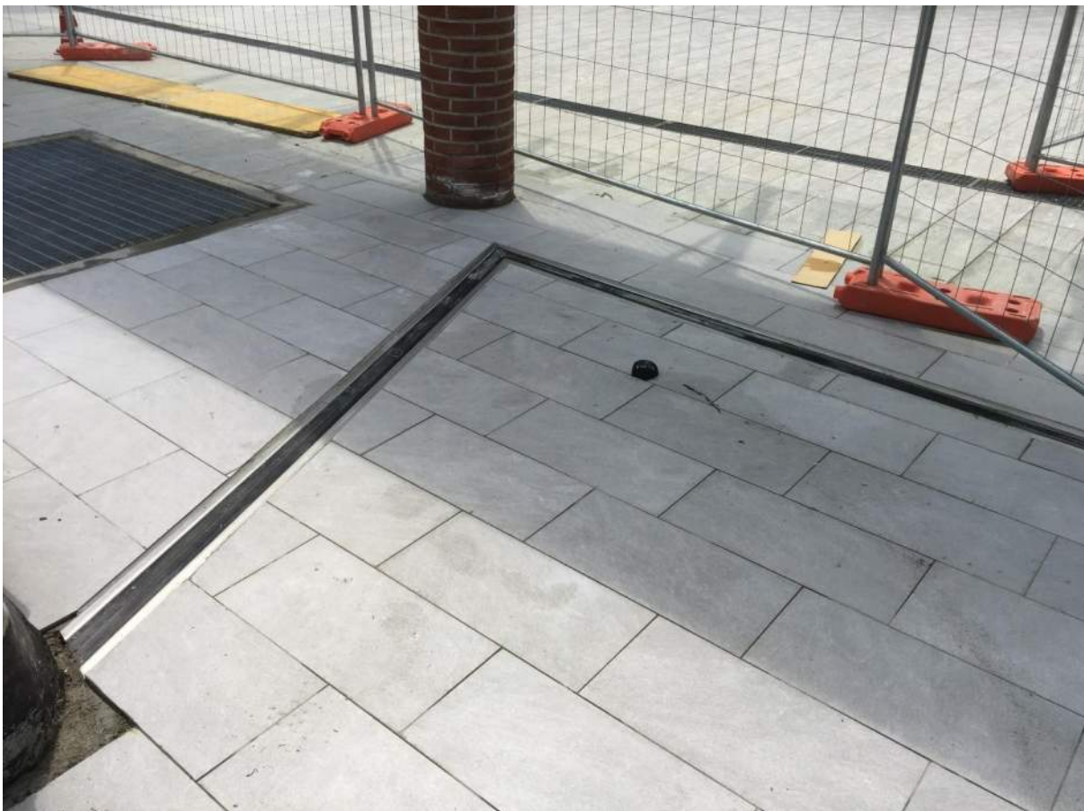
Example of completed movement joint in pavement finishes
