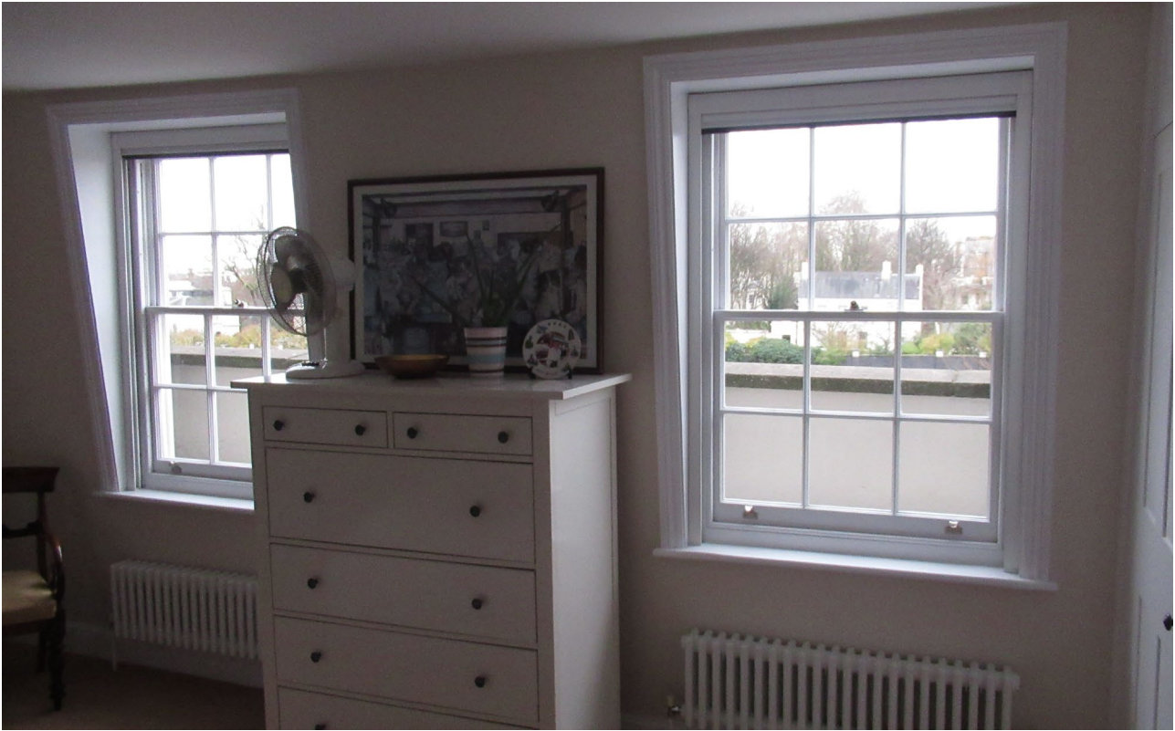
Figure 8: Internal view of 2no. windows in the bedroom at third floor
