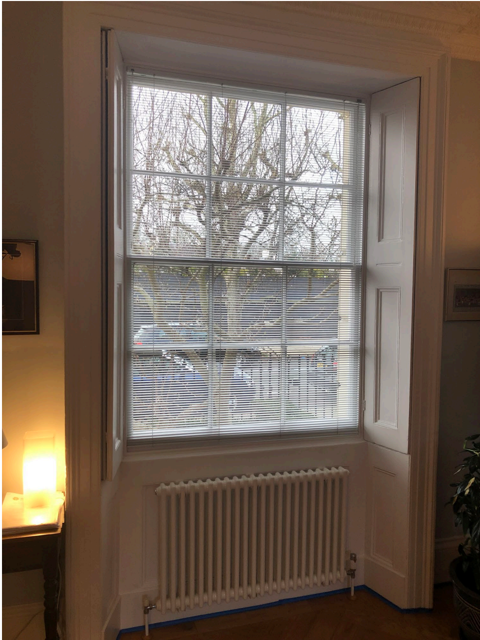
Figure 5: Internal view of window in the living room at ground floor
