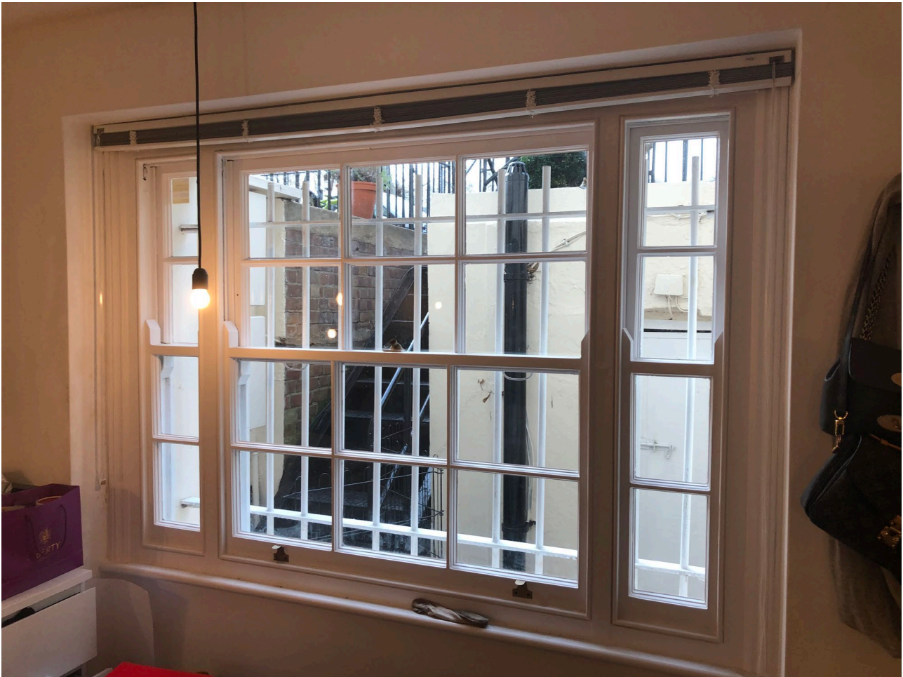
Figure 4: Internal view of window in the living room at basement level
