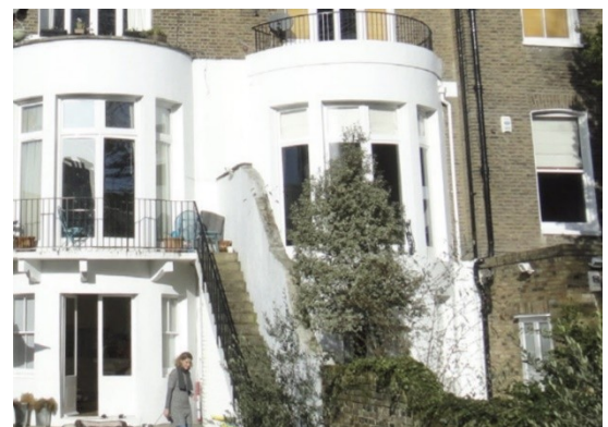
Lower part of rear elevations: No.14- left, No.15- right
