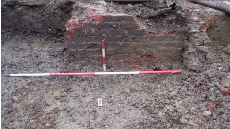
Plate 4: Wall 210, with wall 211 bonded into north face, 2m and 0.40m scales. Looking south
