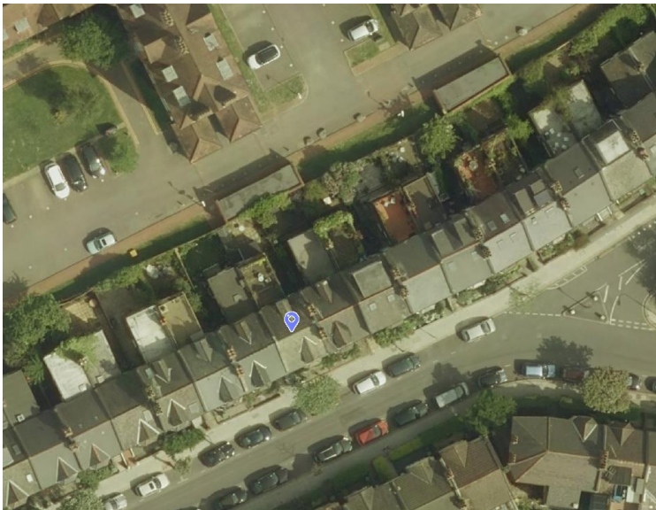
Figure 3 (above): Aerial view of site showing rear roof terrace in situ, dated 2014
