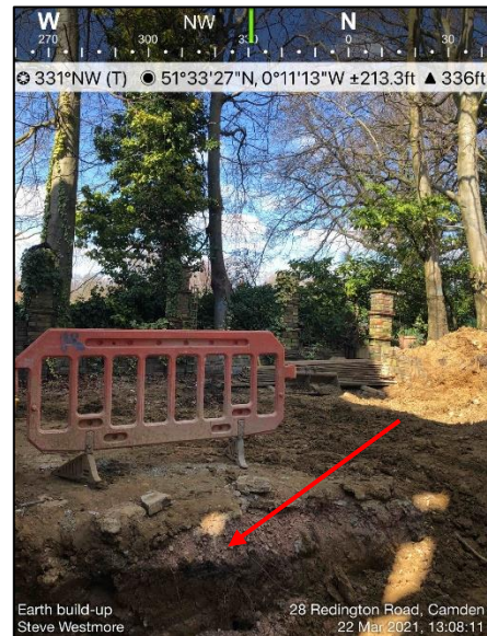
Plate 4 - Soil introduction adjacent T7-T11 with evidence of existing subbase (red arrow)
