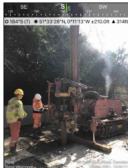
Plate 8 - Piling rig working from on top of temporary ground protection
