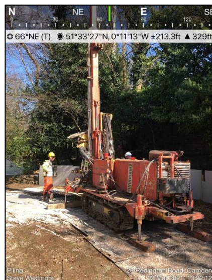
Plate 7 - Piling rig working from on top of temporary ground protection
