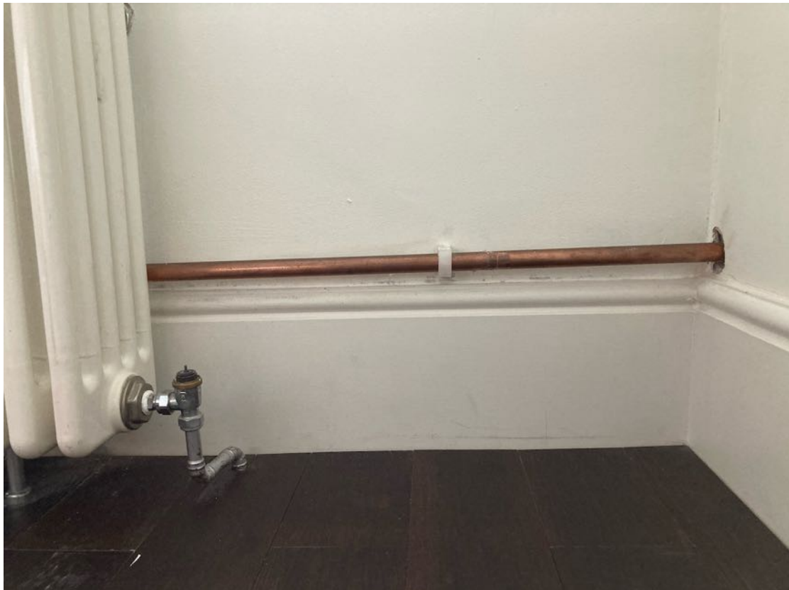
Gas pipe entering Bed 1 through wall from Bed 2.
