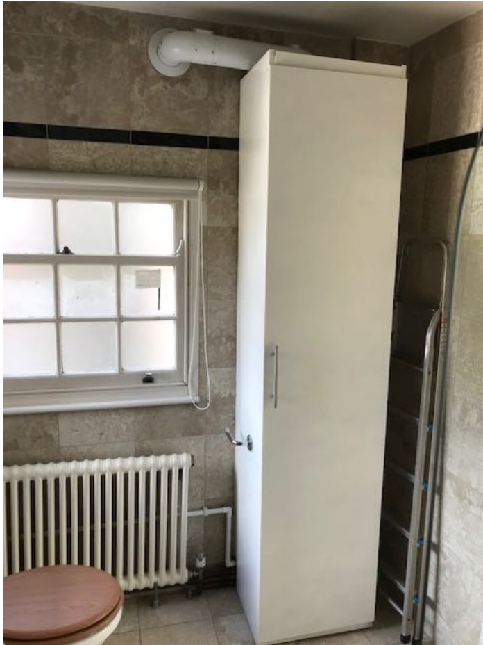
Bathroom boiler cupboard with flue above.
