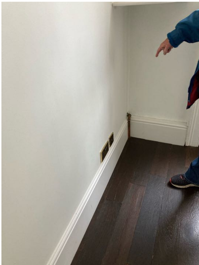
Gas pipe entering Bed 2 from services cupboard at ground floor.
