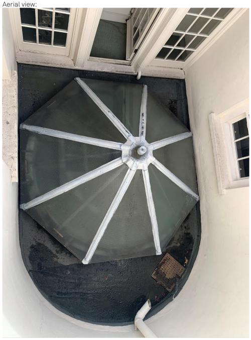
1.2 Existing roof finish around skylight upstand showing poor condition of felt:
