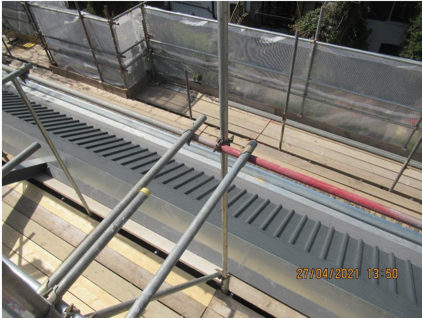
Photographs of new roof to Workshop A
