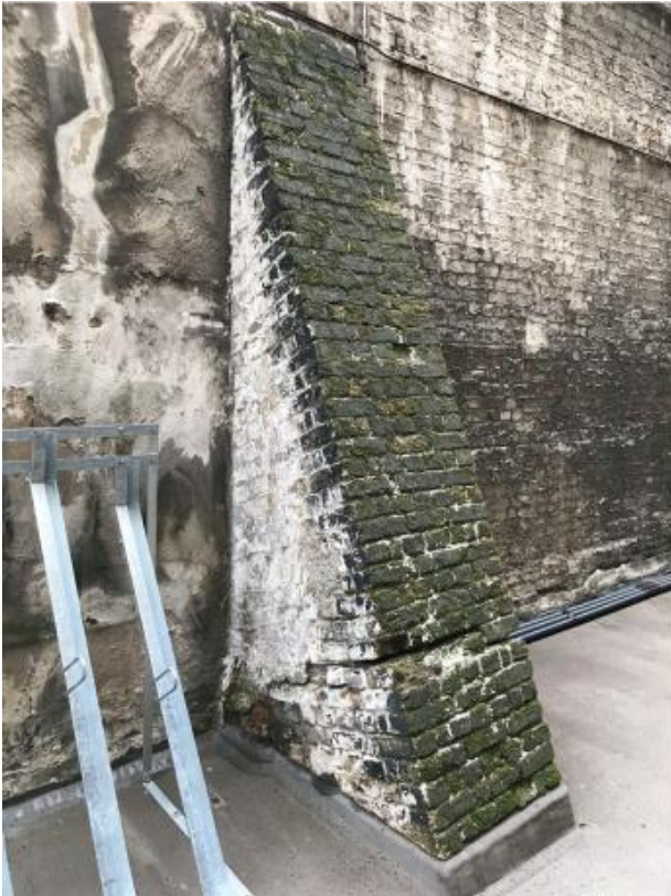
Fig.6, Buttress C : Severe Cracking and separation
