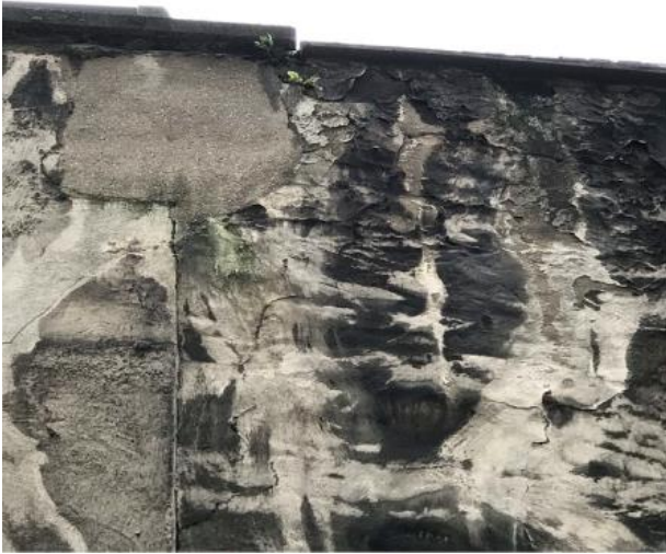
Fig.4, Top of Wall : View onto No 25 & No 24 Ely Place Rear Wall top section illustrating previous remedial localised works
