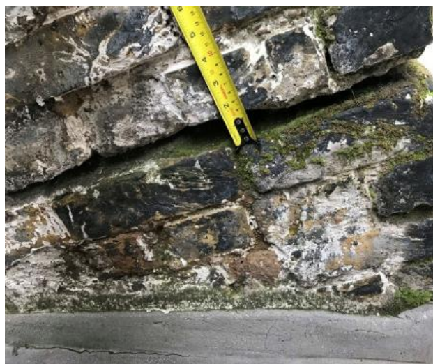
Fig.3, Buttress B : Left Side View, large base crack
