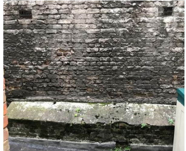
Fig.7, 22 Ely Place : View of damage and wear at the bottom of the wall
