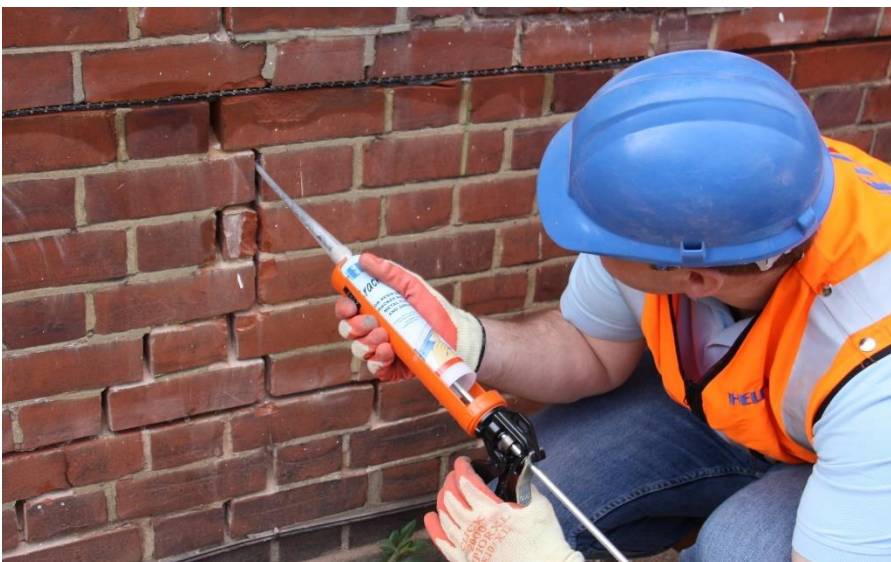
Fig 9. Helifix Resin Crack Repair Stitching Products to Stabilise Cracked Masonry
