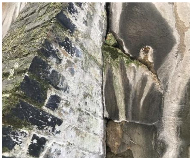
Fig.2, Buttress A : Cracking at the junction with the wall
