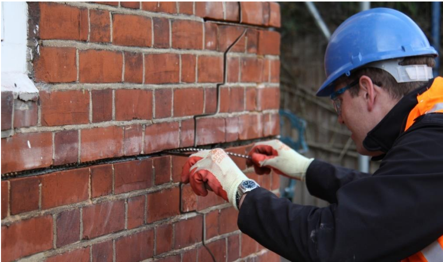
Fig.8 HeliBar (Helifix) Crack Repair Stitching Products to Stabilise Cracked Masonry
