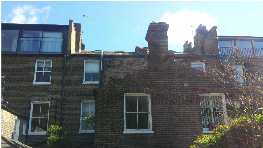
Rear view including existing roof extensions of neighbours' houses to both sides
