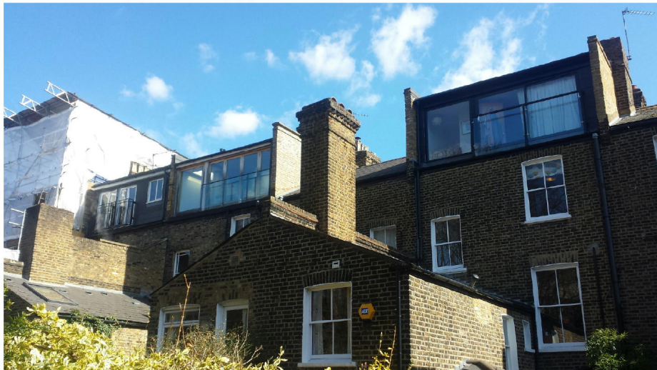
Rear view including existing roof extensions of neighbours' houses to the north side
