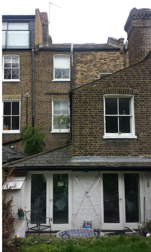
View of Rear Elevation
