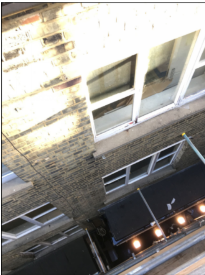
Photo 3 (above): Close-up view of rear elevation windows to be replaced
