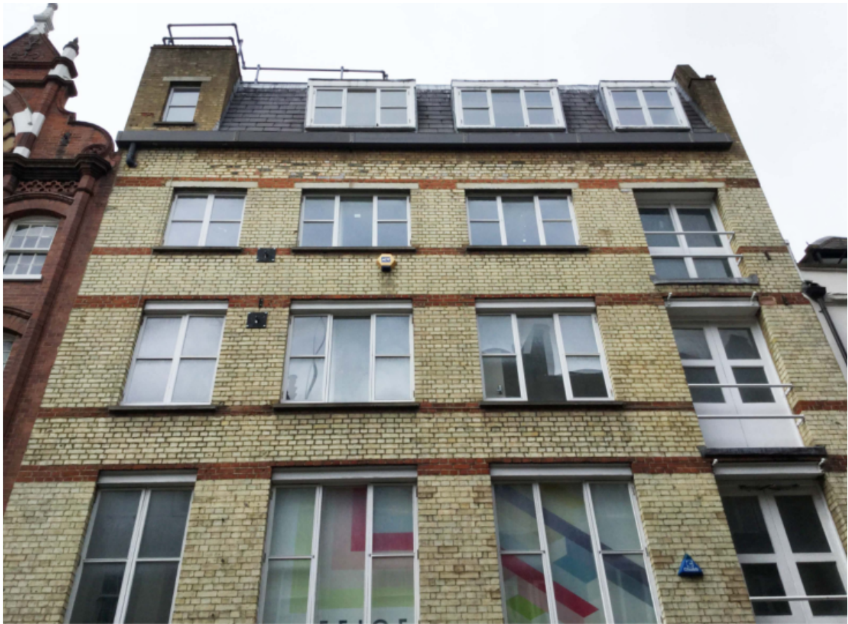
Photo 2 (above): Close-up Front Elevation of Upper Storeys of 57-59 Neal Street
