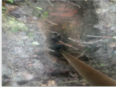
Fig 7.2: Trial Hole 3 Footing
