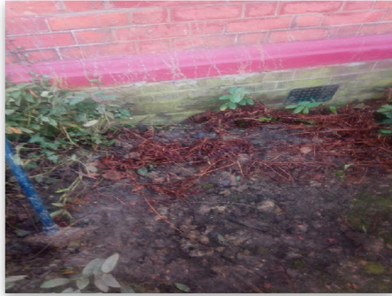
Fig 7.1: Trial Hole 3 Location
