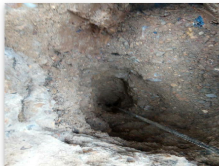
Fig 2.2: Trial Hole 2 Footing
