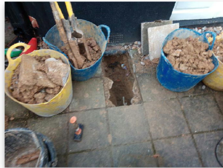
Fig 1.2: Trial Hole 1 Footing
