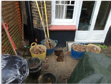
Fig 1.1: Trial Hole 1 Location
