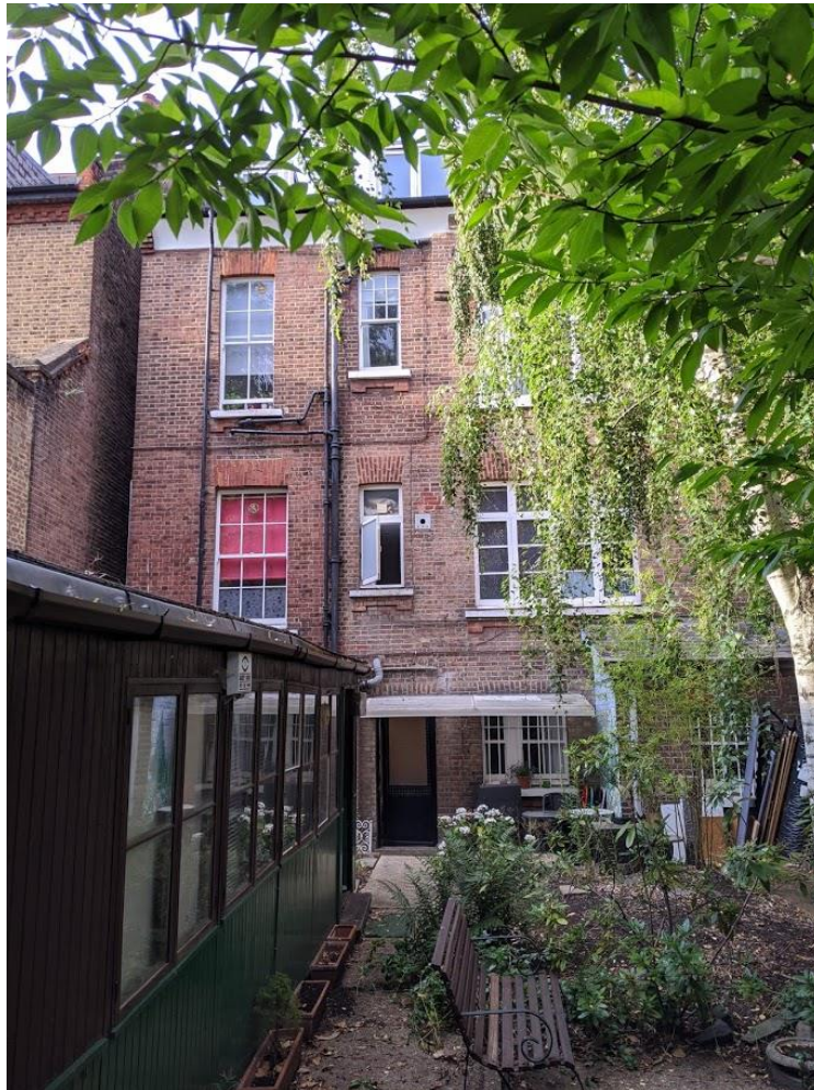
Garden view looking back at 33 Broadhurst Gardens. No 33a is visible to the left. Located within the land of Flat 5, 33 Broadhurst Gdns.
