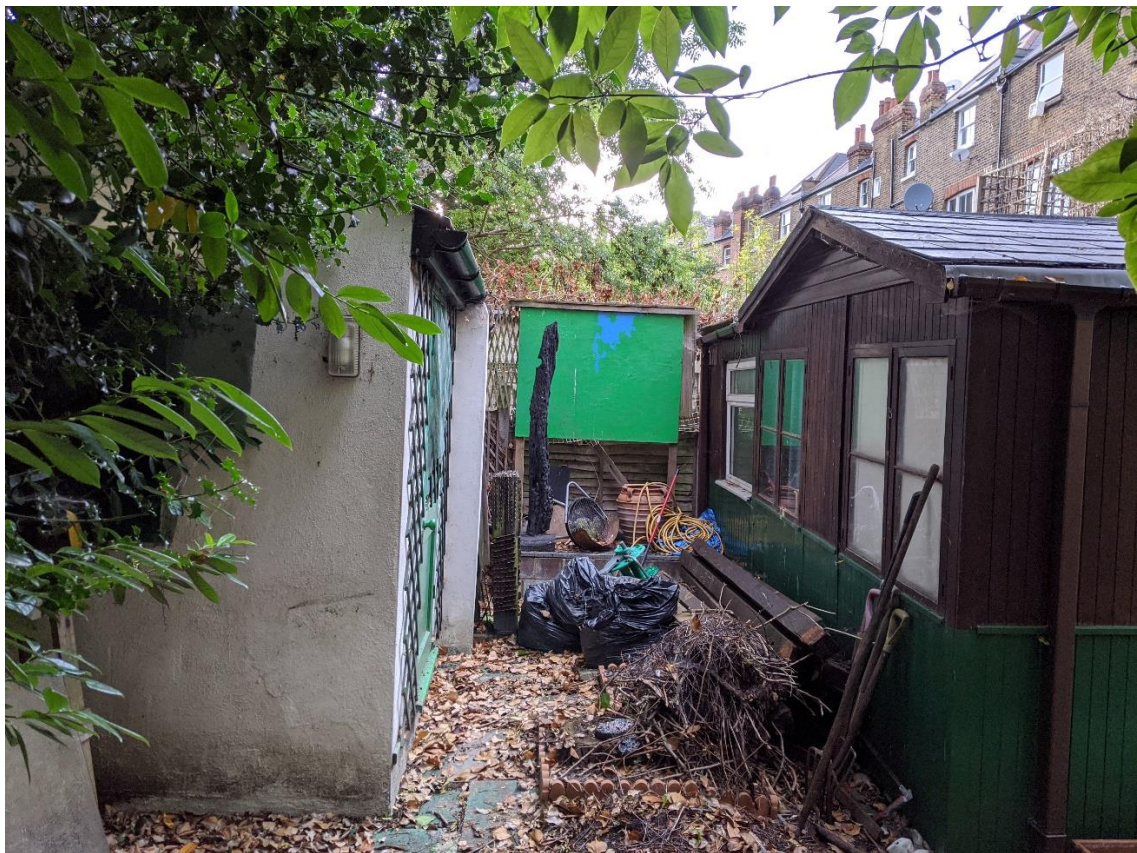
Rear of 33a and brick built garden room to the left.
