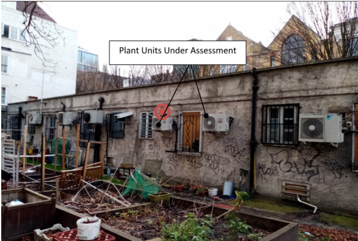
2. Rear elevation showing 2 x plant units
