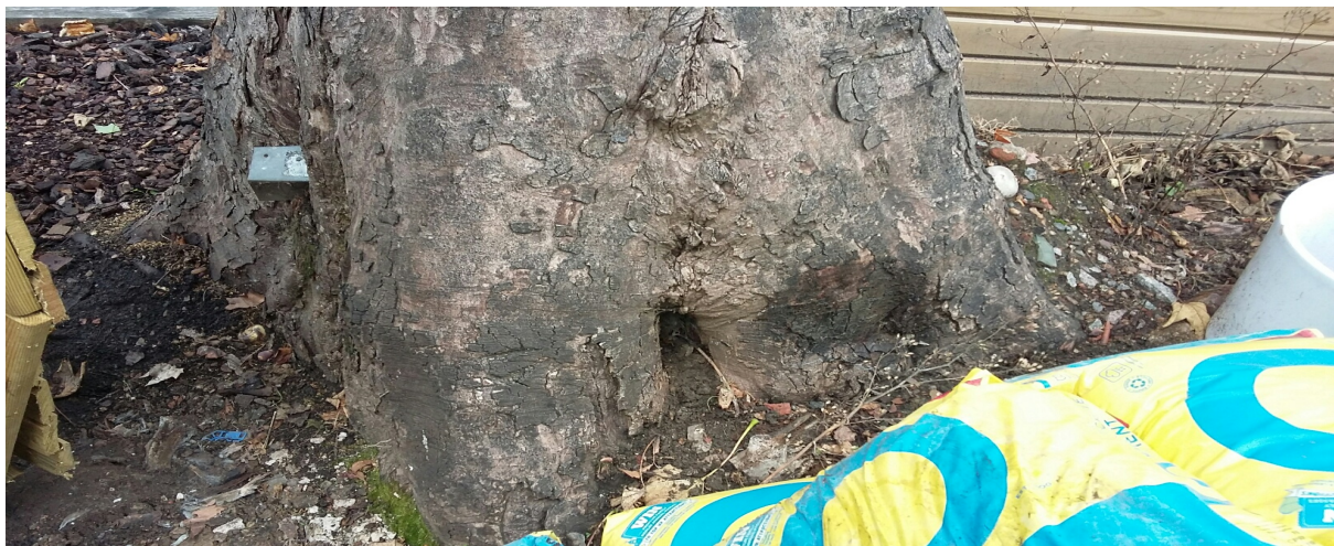
Photograph 2: Small cavity at base of tree
