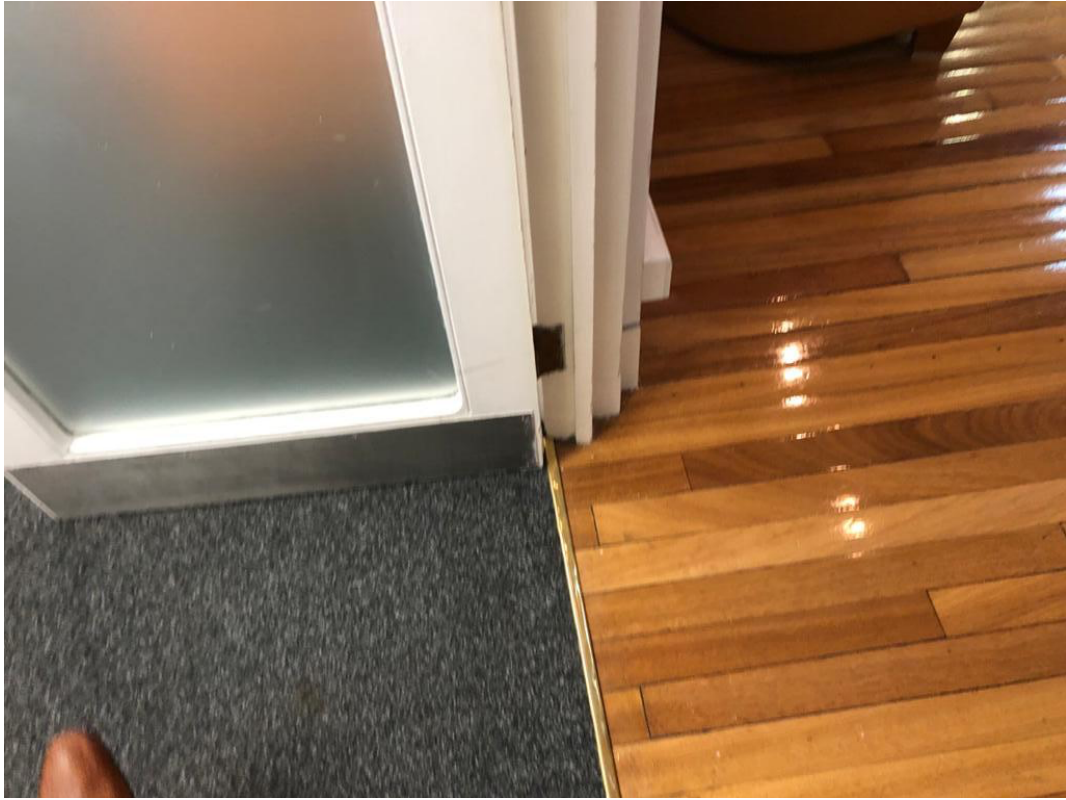
IMAGE 4 – Existing Floor Finish Transition between Syndicate Room and Lift Lobby
