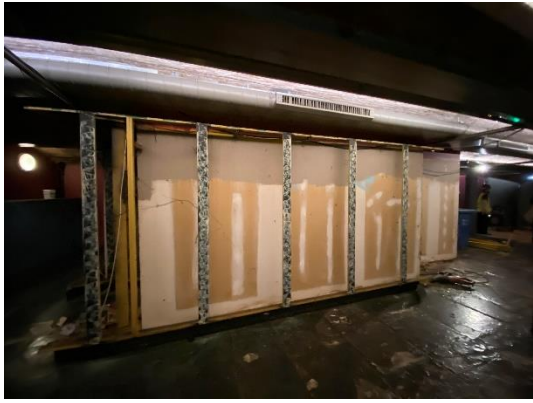
5. Glass wash and chillers
