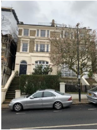
House frontage & T's 1 & 2
