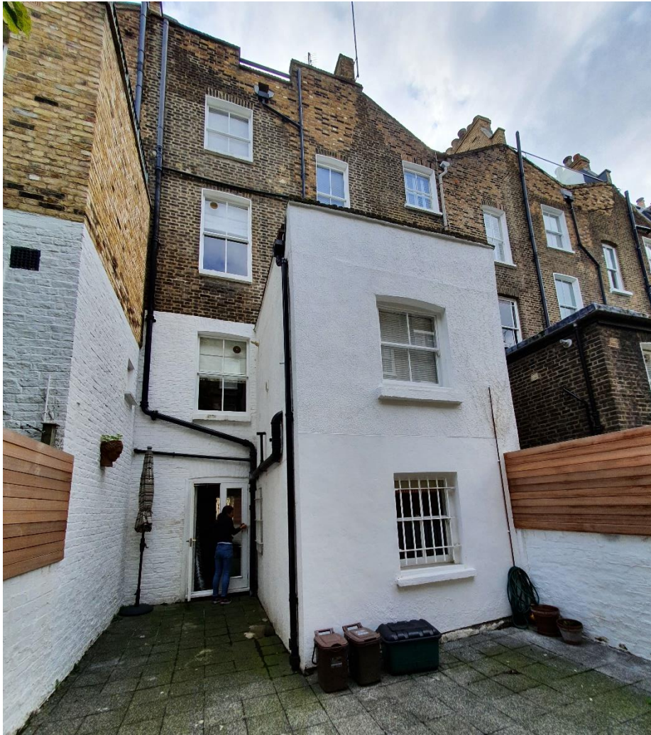
Image 8. Rear view (North Elevation) of 55 Princess Road.
