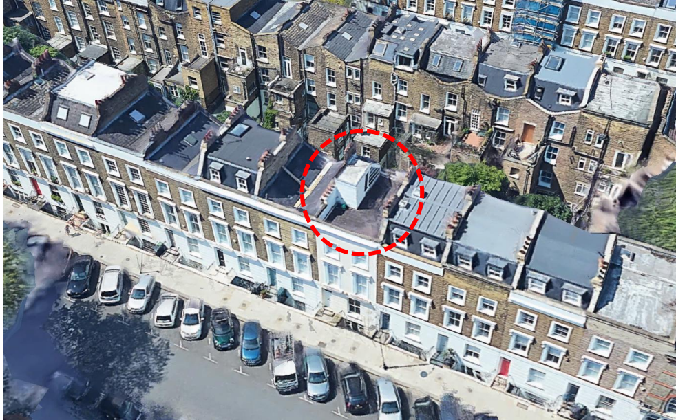
Image 9. Aerial view of 55 Princess Road.
