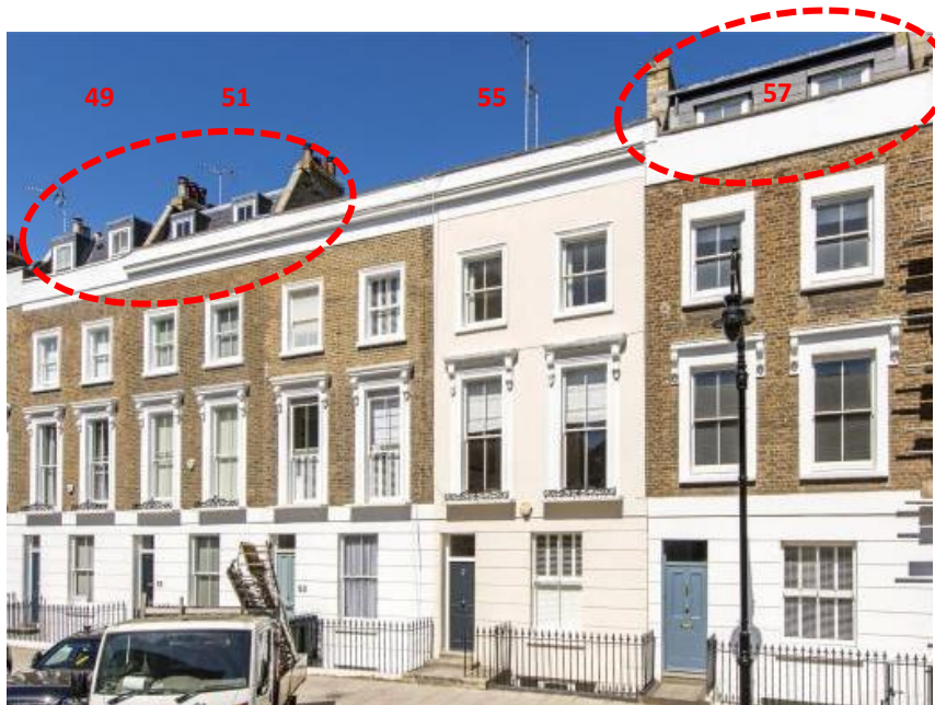
Image 10. Mansard roof developments on Princess Road.
