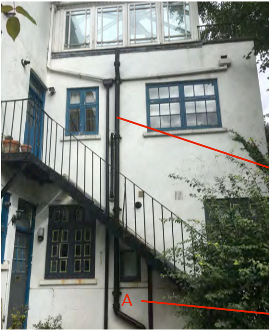
propped landing meets top of stairs that run across facade.
