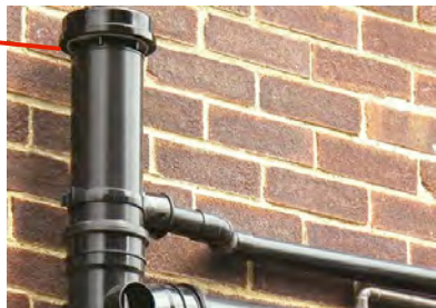
example of a standard AAV termination
