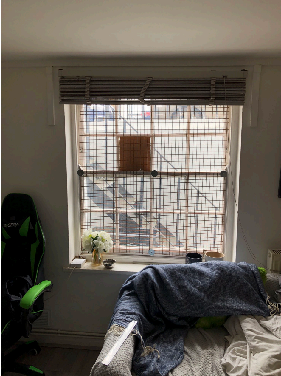
Figure 6: Internal view of window in lounge at basement level
