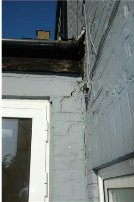
Separation cracking rear outrigger with two storey section
