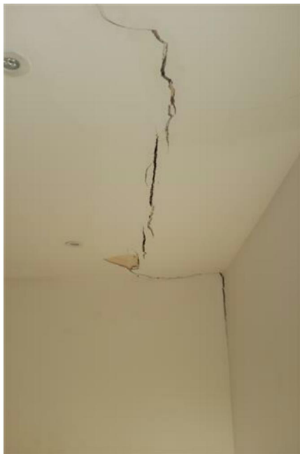
Cracking in ceiling at junction of rear outrigger with main
