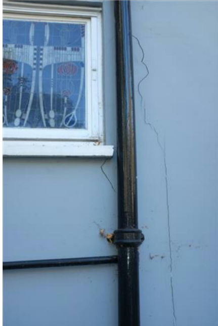
External cracking front right hand side of two storey section
