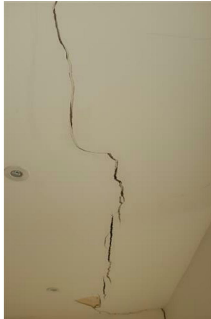
separation cracking in ceiling in rear outrigger
