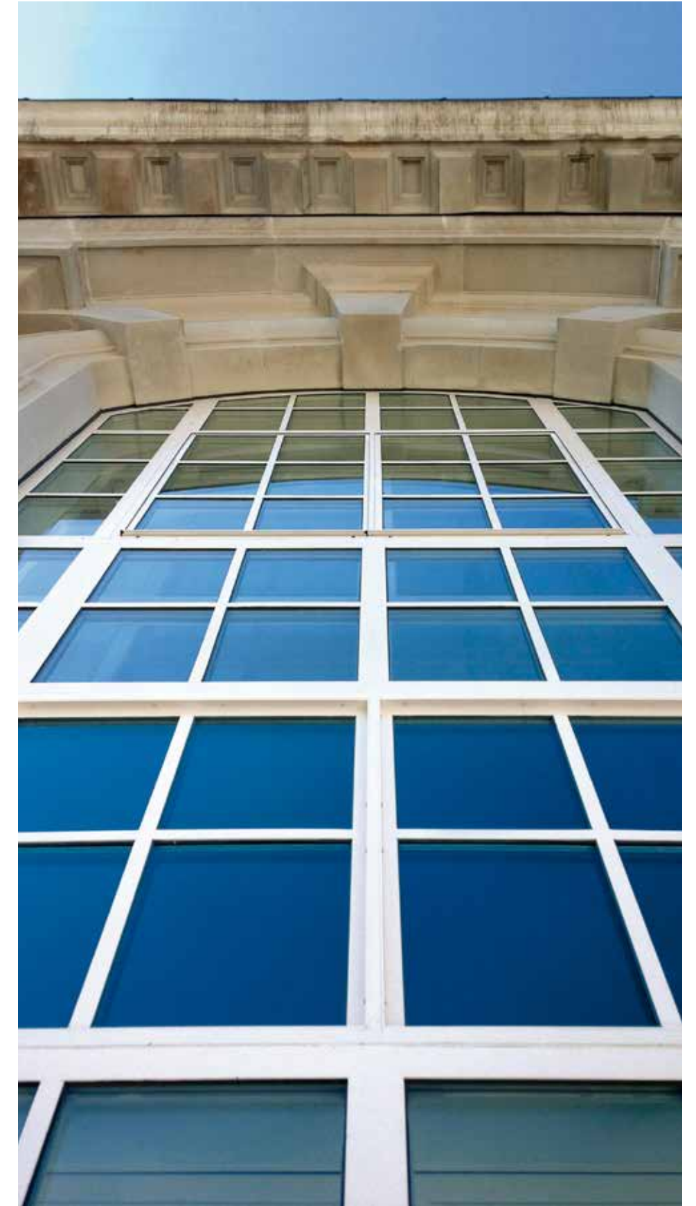
04. Close up of Janson Janisol Arte 2.0 windows installed on Regent Street, London borough of Westminster.
