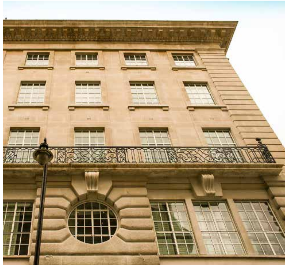
01. Example of Janson Janisol Arte 2.0 windows installed on Regent Street, London borough of Westminster.
