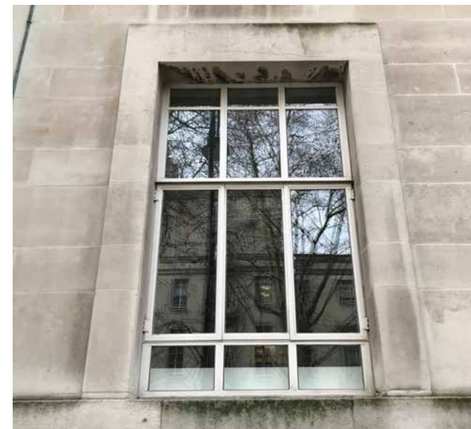
04. Typical single-glazed non-thermally broken steel (installed 1995-2000) found on Malet Street facade.
