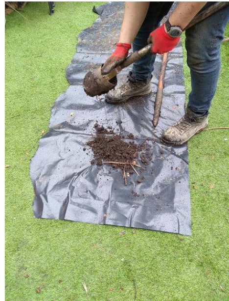
Plate 10: Topsoilly Made Ground encountered.
