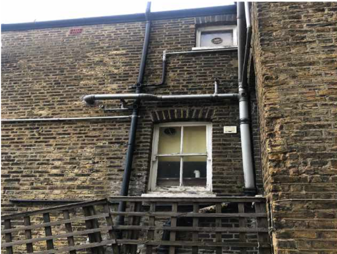
3 - 63 Fortress Road rear extension side windows
