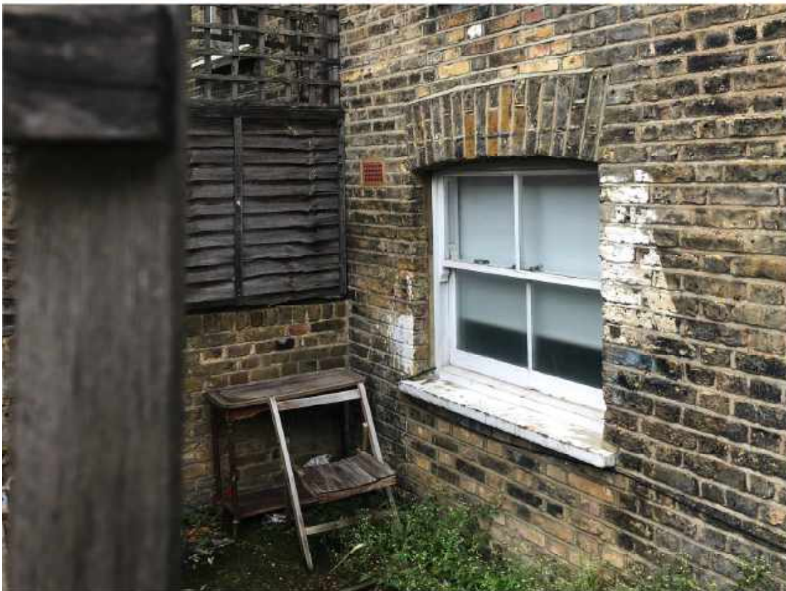
3 - 63 Fortress Road rear extension Lower Ground Floor courtyard window
