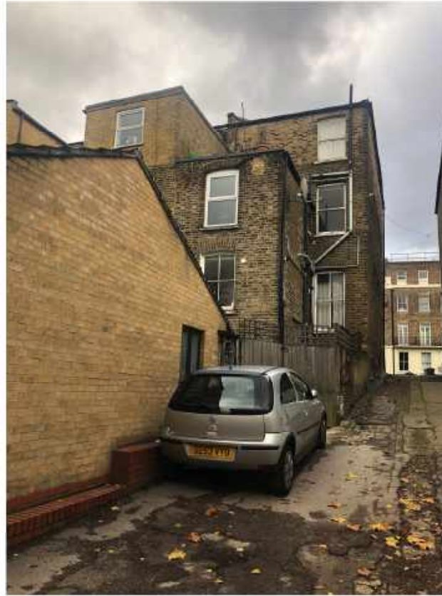
1- 63 Fortress Road Rear Elevation
