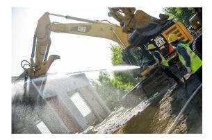
A fire hose will be used for direct suppression during mechanical demolition.
