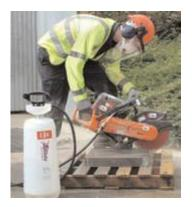
Proprietary water suppression will be used on all cutting devices.
