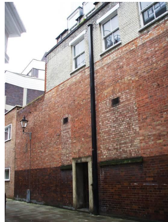
Flank elevation to the passageway
