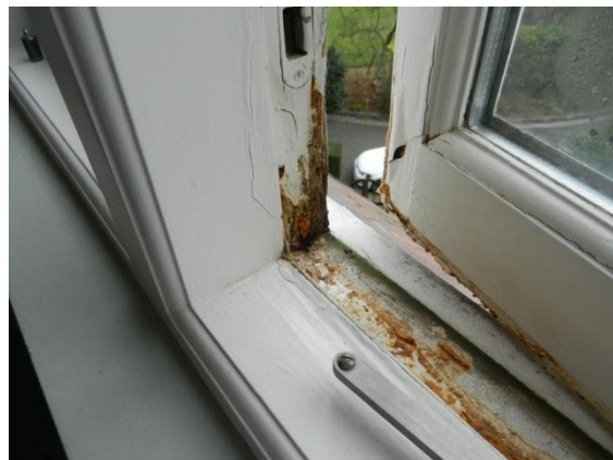
Fig. 12 Rotten 2 nd Floor Window.
