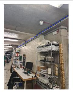
New cable to be installed alongside the path of the existing cable along the roof as indicated above.
