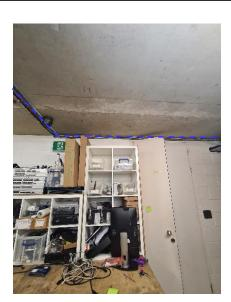
New cable to be installed alongside the path of the existing cable along the roof as indicated above, before turning at the wall and running past the communications room.
