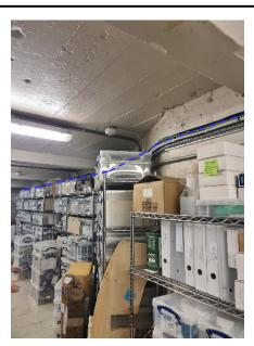
New cable to be installed alongside the path of the existing cable along the roof as indicated above.
