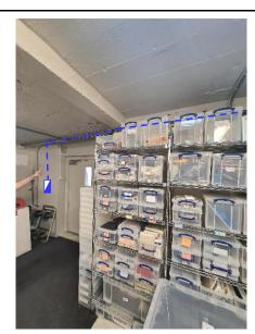
New cable to run from the BFP above the door (following the path it entered) where it will then follow the path of the existing cable as indicated above.
