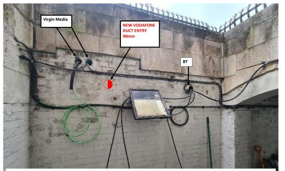
Core drill basement well area and install new 90mm duct entry. Rope and seal duct once installed. (positioned on same wall next as other telecoms providers duct entries)
