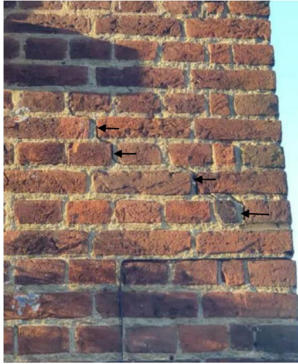
Stepped cracking to front elevation
