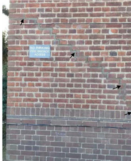
Stepped cracking to right hand side elevation
