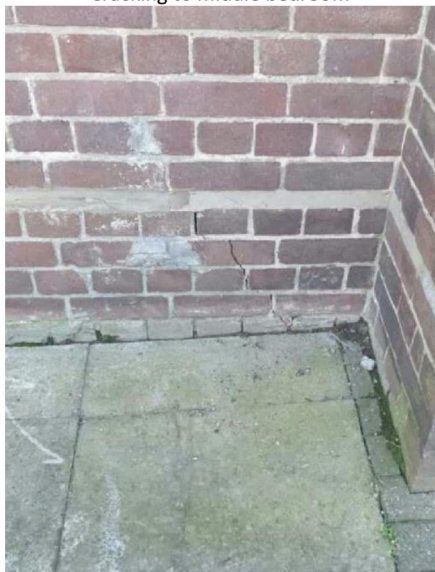
Cracking to right hand side
