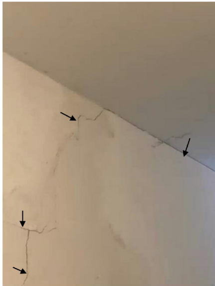
Cracking to middle bedroom
