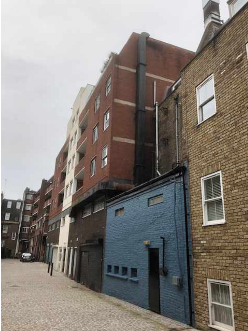
View south along Fitzroy Mews towards building
