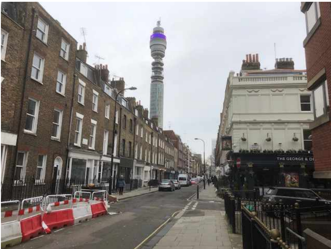
View south along Cleveland Street towards building
