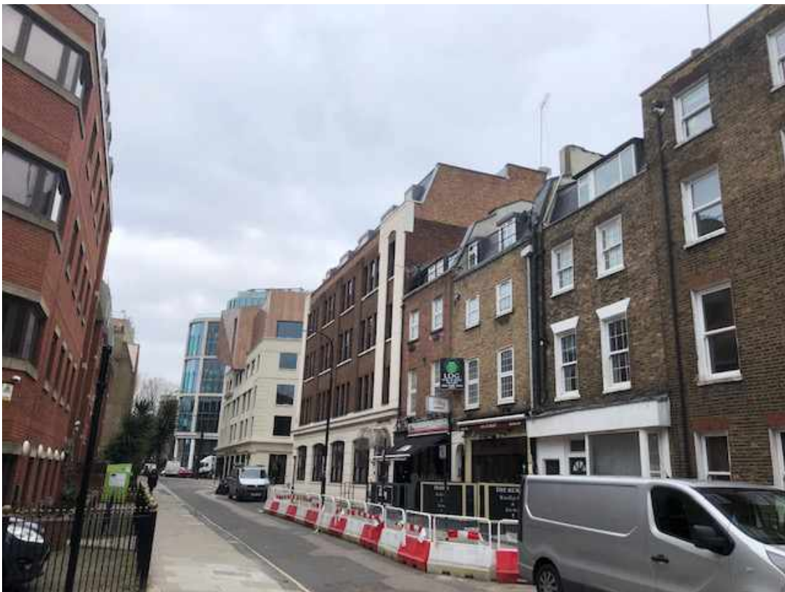
View of copper clad two storey addition on Cleveland Street / Warren Street
