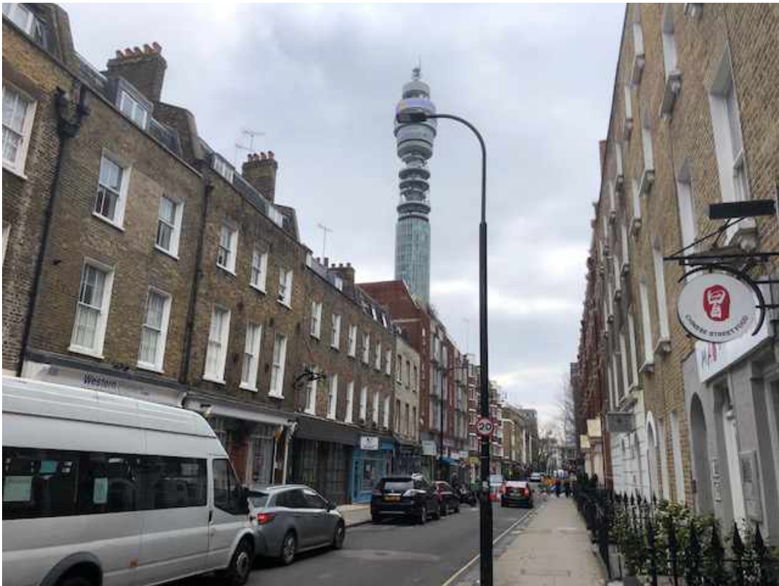
View south along Cleveland Street towards building
