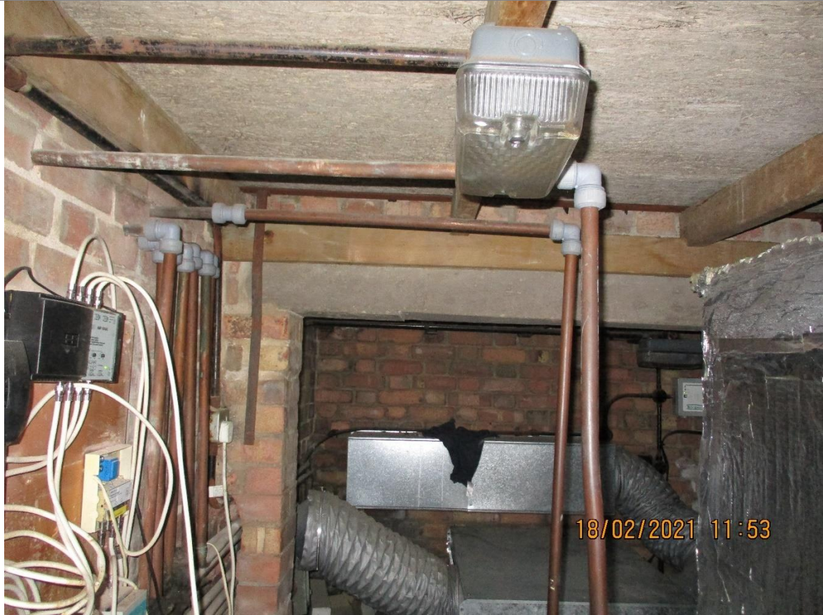
Photograph 6: Lift Motor Room - showing brick and concrete structure
