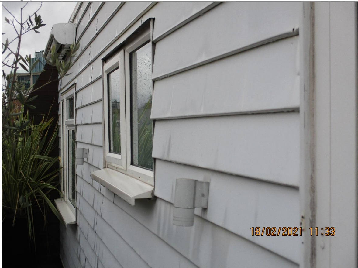
Photograph 5: Top Floor east & west elevations
