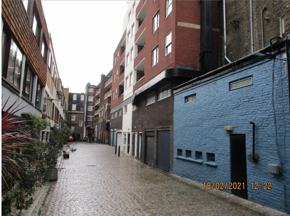
Photograph 2: Fitzroy Mews Elevation - note slope
