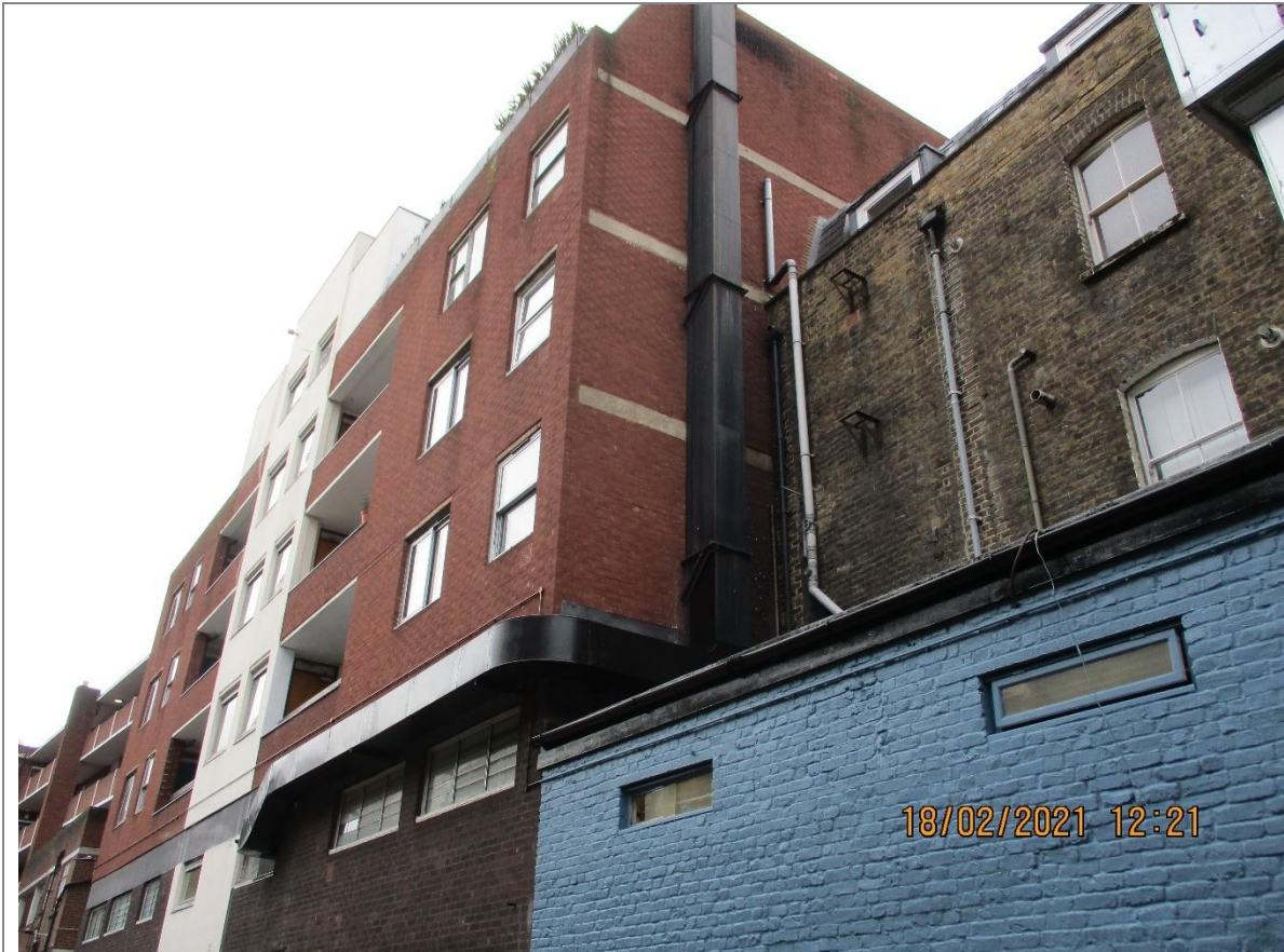
Photograph 4: North elevation - note slab levels
