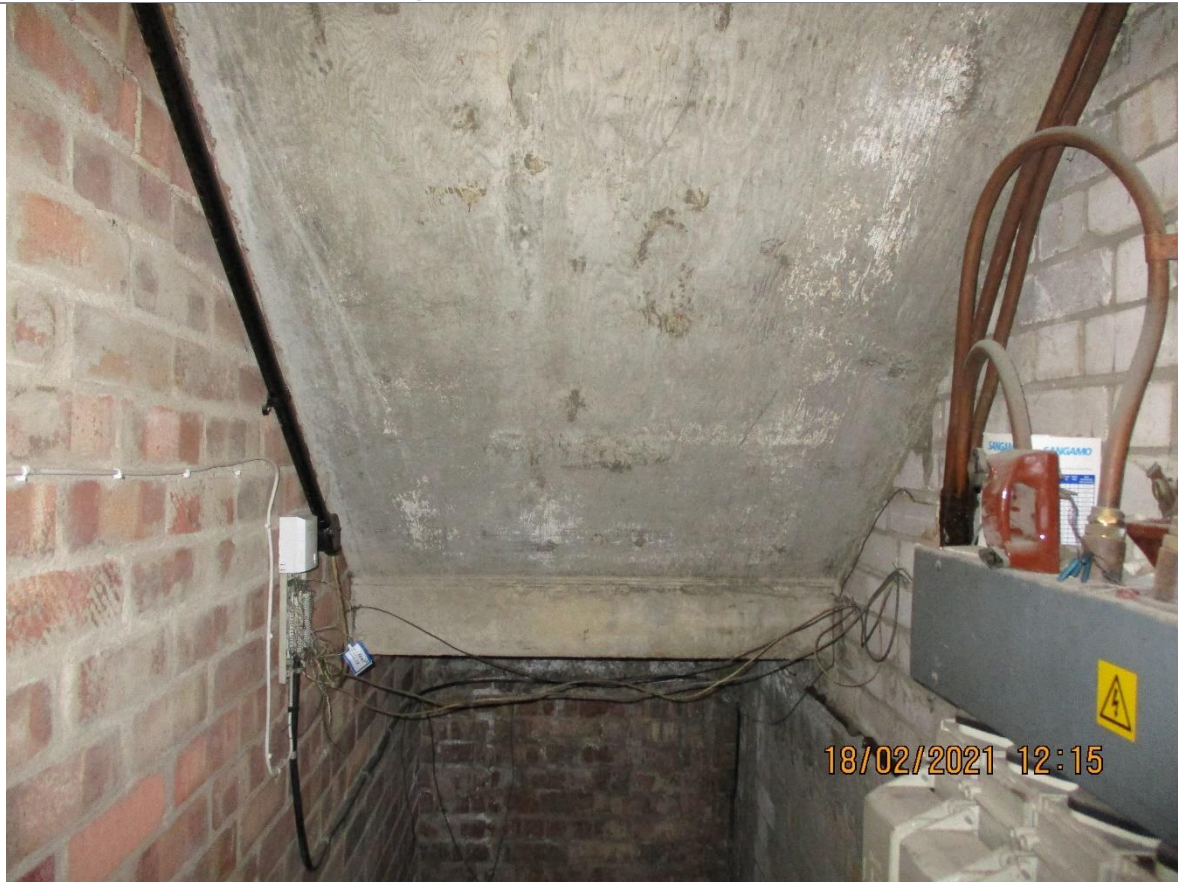
Photograph 7: Undercroft showing brick and concrete construction
