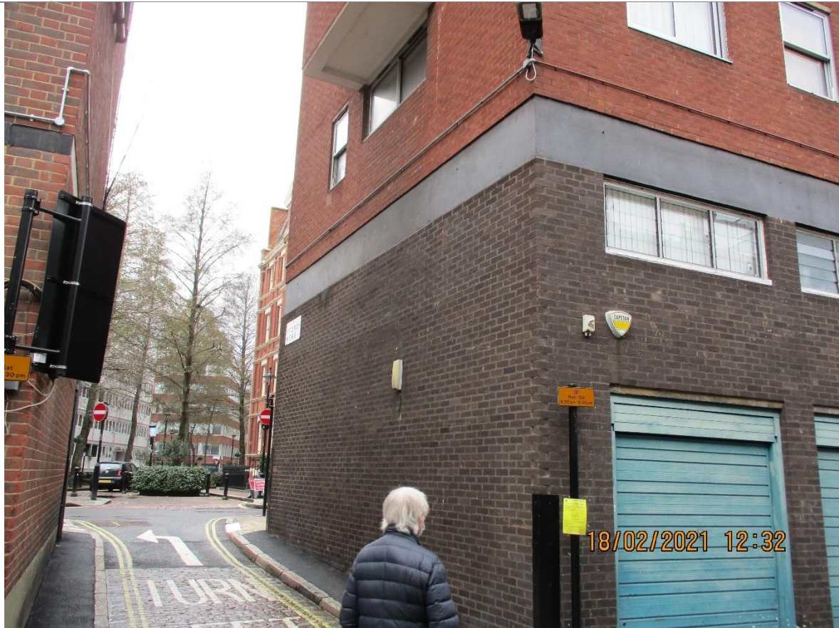
Photograph 3: South Elevation - note slope
