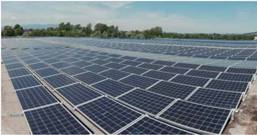
Slovenia Installation: 150 kW | S-Dome System
