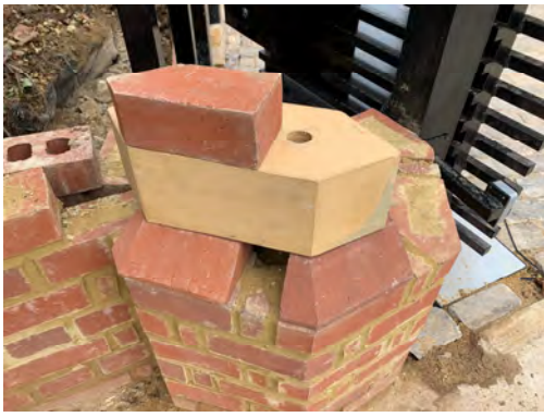
11. Pier adjacent to No18 showing replacement crease, terracotta band and replacement brick, Saxon Red Multi.
