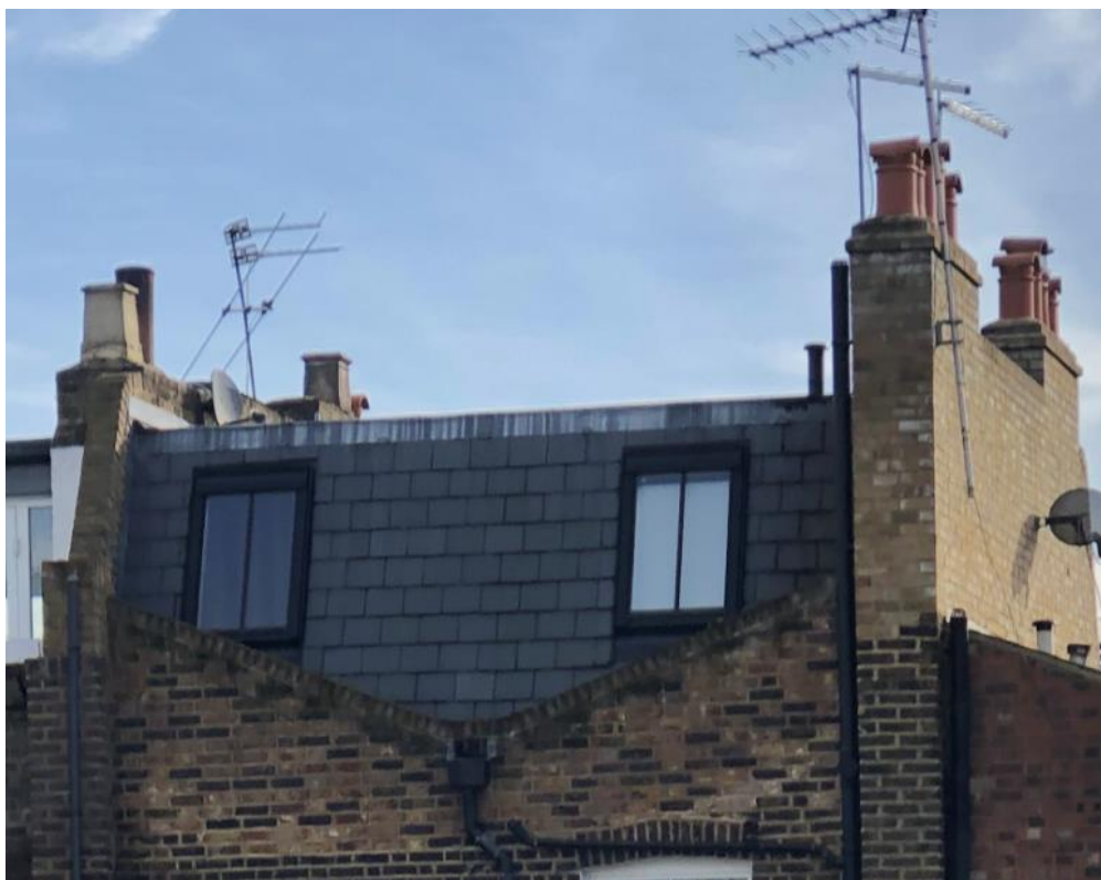
Fig. E Rear parts of a property on Egbert Street as viewed from the rear terrace of 17 Fitzroy Road. The proposal at 17 Fitzroy will match this style of mansard, rooflights, V shaped parapet and drainage.
