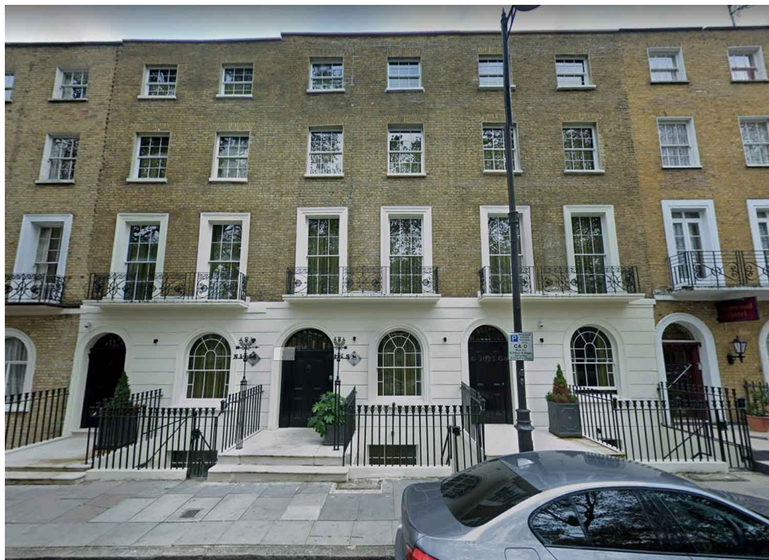
No.16, 17, 18 Argyle Square reinstated original sash windows on all front elevations
