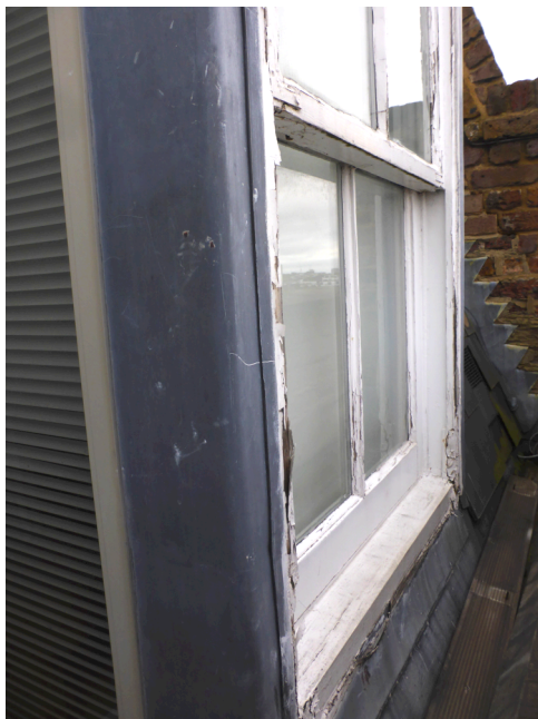
Figs. 2 & 3 existing rotten timber sash windows clad with zinc; inset front terrace with glazed returns and sliding glazed doors
