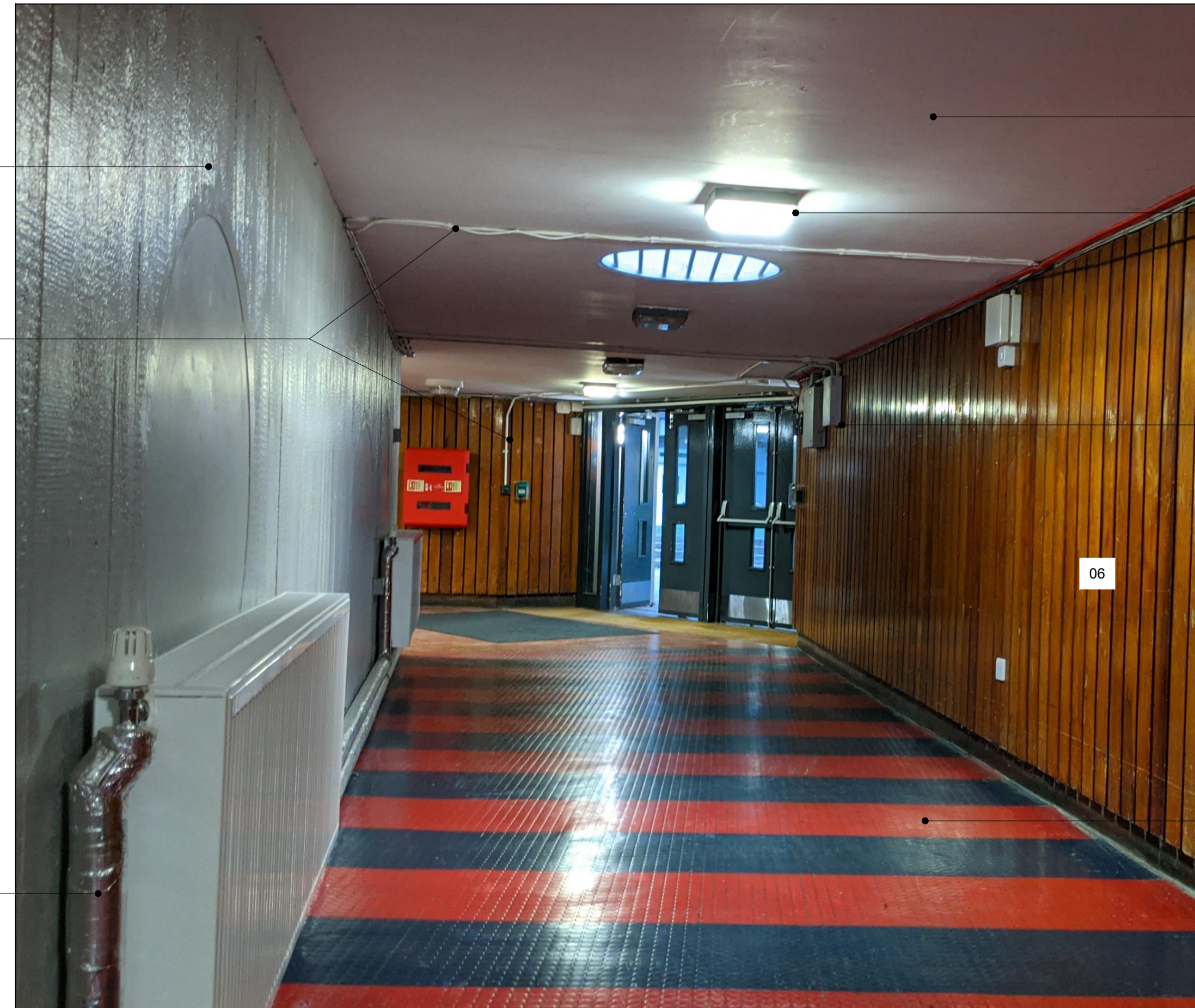
2. CORRIDOR LOOKING TOWARDS MAIN ENTRANCE
