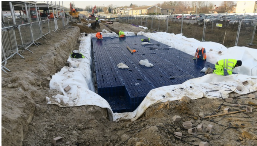
Figure 6 Below ground geo-cellular attenuation tank
