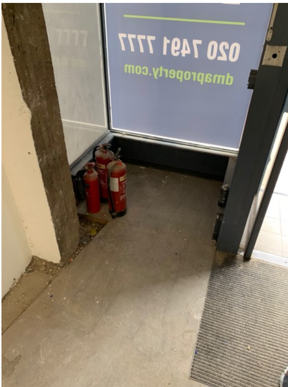
Existing shop front internal view, 02
