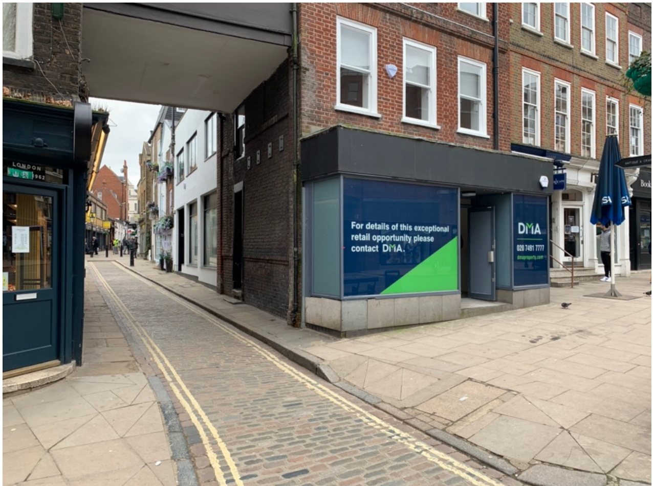
72 Hampstead High Street, external view from the high street
