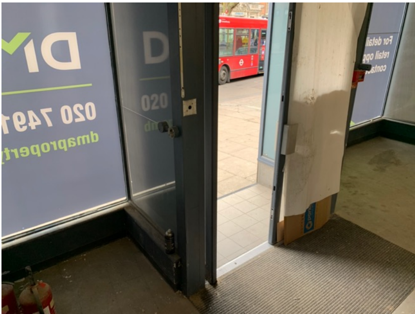
Existing shop front internal view, 04
