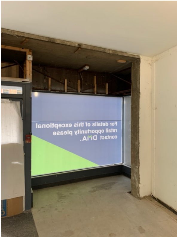
Existing shop front internal view, 01
