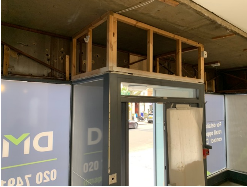
Existing shop front internal view, 03, showing concrete slab above
