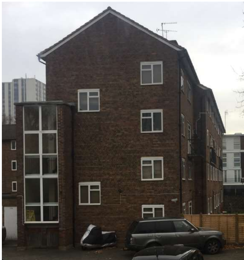
Image 5 – 106 Hawtrey Road and 3 Lyttelton Close, north facing elevation
