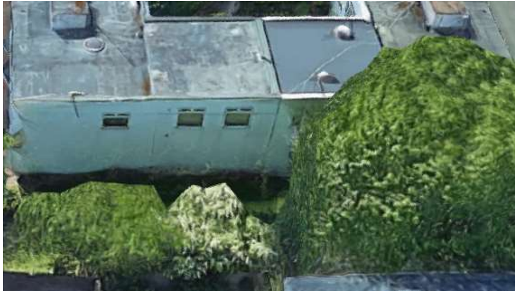
Image 4 – 3 Lyttelton Close and 106 Hawtrey Road, north facing elevation
