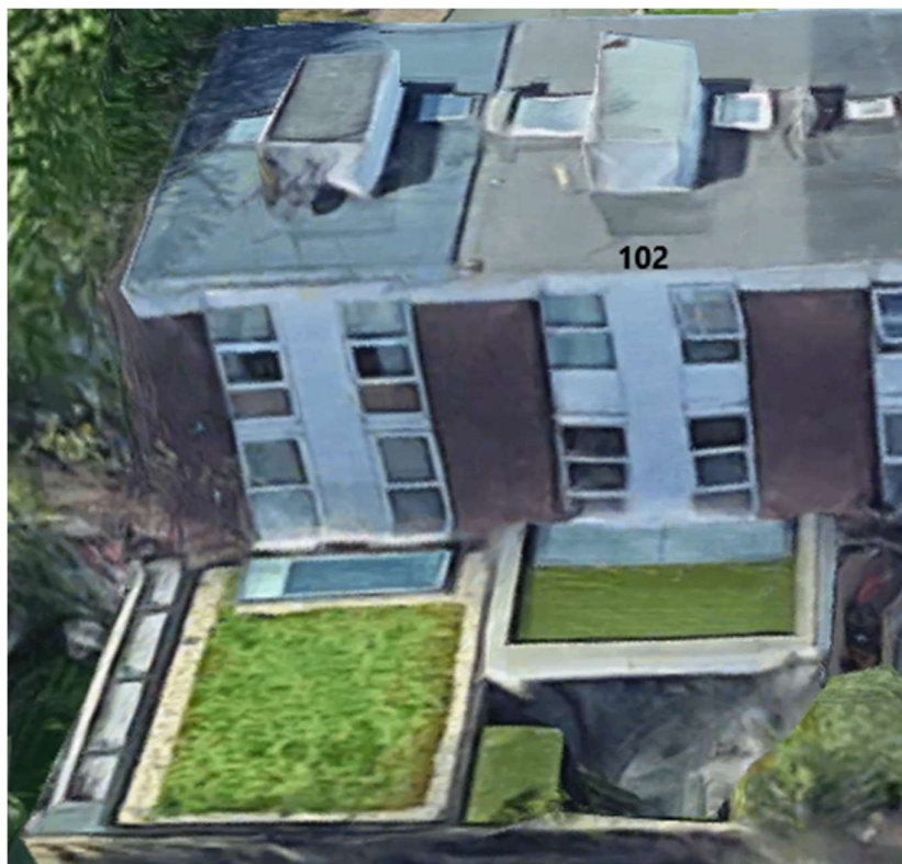
Image 3 – 102 Hawtrey Roader Street, east facing elevation
